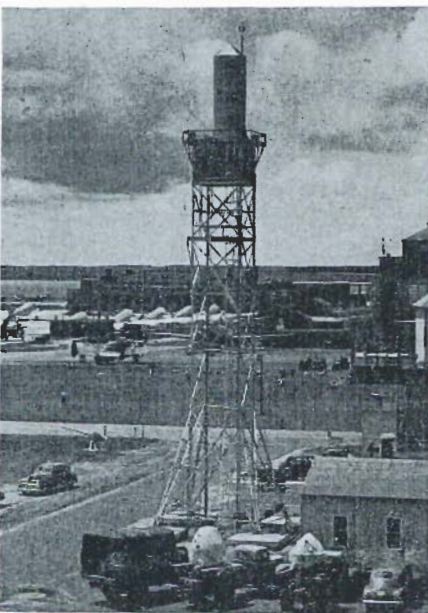
Height-finding antenna supplies data to search operator in control tower
